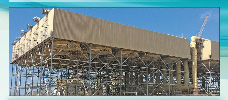
EVAPCO Dry Cooling single row heat exchanger cores are in operation in over 35 power plants with combined electrical generation of over 12GW. This type of heat exchanger core has been in operation worldwide since 1990.
