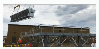
**eco-Air Air Cooled Heat Exchangers**Easy Installation of Factory Assembled Packaged Units
