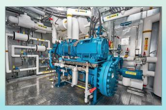
Evapcold Low Charge Ammonia Machinery Room LCR-P-W
