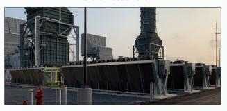
**eco-Air Air Cooled Heat Exchangers**Factory Assembled Packaged Units Located at Grade
