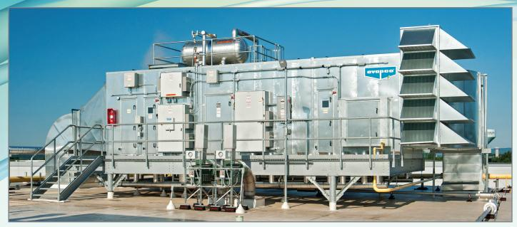
Critical Process Air (CPA) Hygienic Air Handling System
