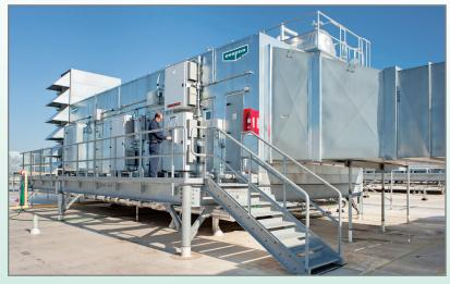
Critical Process Air (CPA) Hygienic Air Handling System
