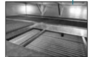
and debris buildup. Type 304 or 316 stainless steel is available to provide increased corrosion protection for the entire basin area including the support columns of the cooler and the air inlet louver frames.
