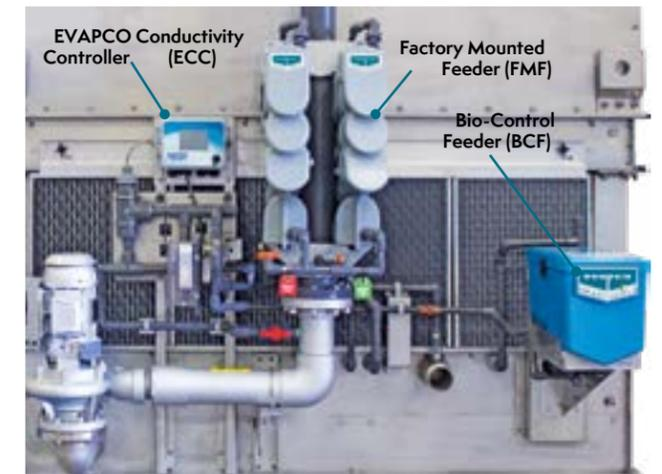
EVAPCO's Smart Shield® system utilizes proven solid chemistry delivered via our revolutionary feed system. With patented Controlled Release tablets, a scale and corrosion inhibitor is fed whenever your spray water pump is energized. Thus keeping your system protected anytime the spray water pump is operating.
