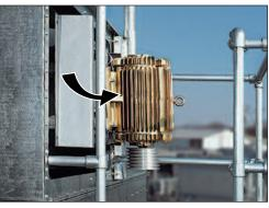
Internally mounted fan motor can swing outside the unit for easy access.
