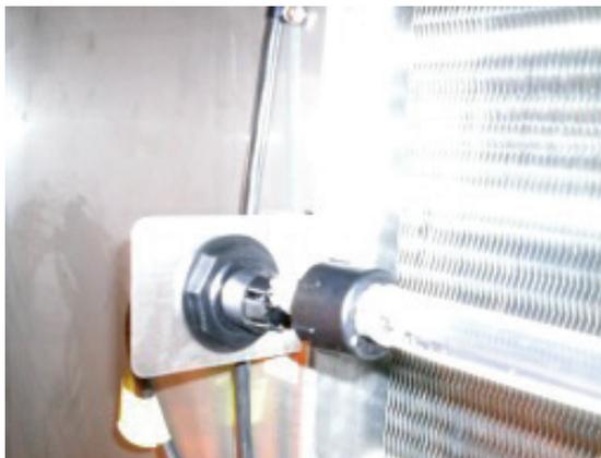
2. Plug the bulb into the four hole socket and make sure it is fully seated. Now slide the ring tight against the assembly and tighten the fitting. **Hand tighten only – never use a tool!** Failure to properly install the waterproof assembly can cause premature failure of the bulb.
