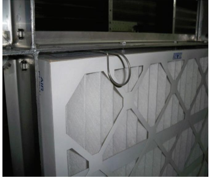
The MERV 14 and 15 final filters are held in place with four spring holding clips or clamps. The MERV 14-15 (95%) filters use a spring clip, fastened to the back flange of the filter frame. Once the filter is installed, the spring clip should be fastened on the plastic part of the filter. All filters should be installed, if possible, with the pleats vertical.
