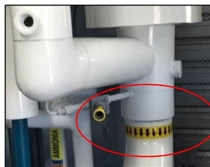
In addition to the oil separation being more effective in the Evapcold design, we have also included a means to return any oil carryover to the compressor via a small 3/8" metering line from a low point in the recirculator to the compressor suction (see photo above). The oil return line is not insulated so any liquid refrigerant will vaporize before entering the compressor.
