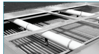
Drift Eliminators Removed for Coil Inspection
