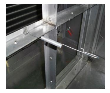
The 99.95% HEPA filters use an angle clip that fits in a notch in the frame.
