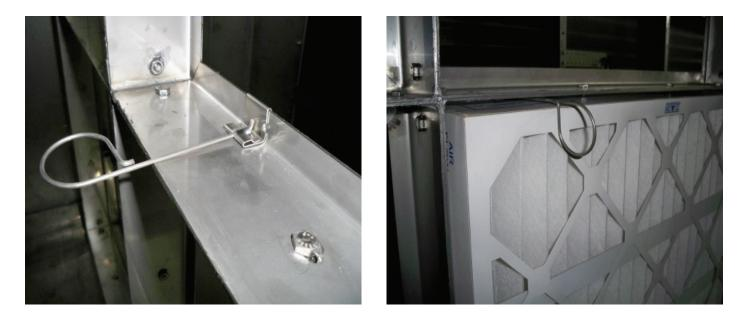
The MERV 14 and 15 final filters are held in place with four spring holding clips or clamps. The MERV 14-15 (95%) filters use a spring clip, fastened to the back flange of the filter frame. Once the tilter is installed, the spring clip should be fastened on the plastic part of the filter. All filters should be installed, if possible, with the pleats vertical.
