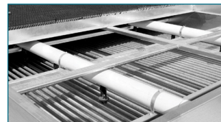
Drift Eliminators Removed for Coil Inspection
