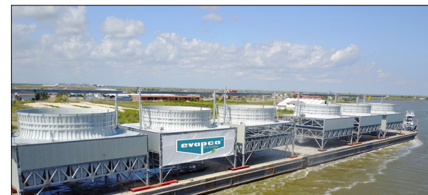
Advanced Technology™ ACC Offsite Modularization
