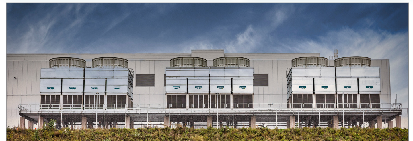
AT Atlas installation
