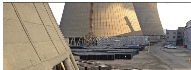
Major projects/Natural draft refurbishments
