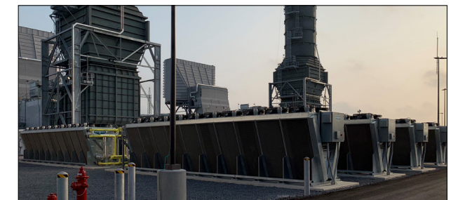
eco-Air Air Cooled Heat Exchangers Factory Assembled Packaged Units Located at Grade
