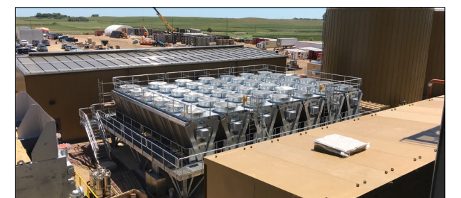
eco-Air Air Cooled Heat Exchangers Factory Assembled Packaged Units Installed on Common Structure
