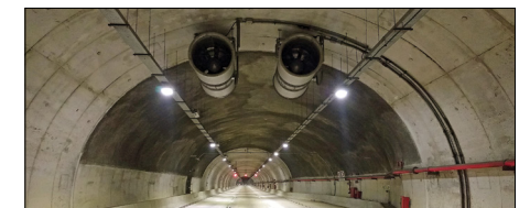
Road Way Ventilation System – FRP High Temperature Class
