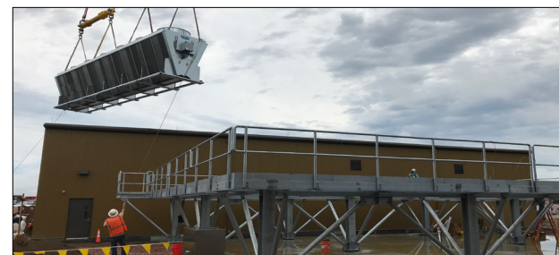
eco-Air Air Cooled Heat Exchangers Easy Installation of Factory Assembled Packaged Units
