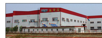
EVAPCO (Beijing) Refrigeration Equipment Co., Ltd, Beijing, China
