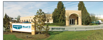
EVAPCO Alcoil, York, Pennsylvania
