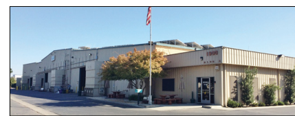
EVAPCO West, Madera, California
