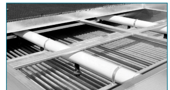
Drift Eliminators Removed for Coil Inspection
