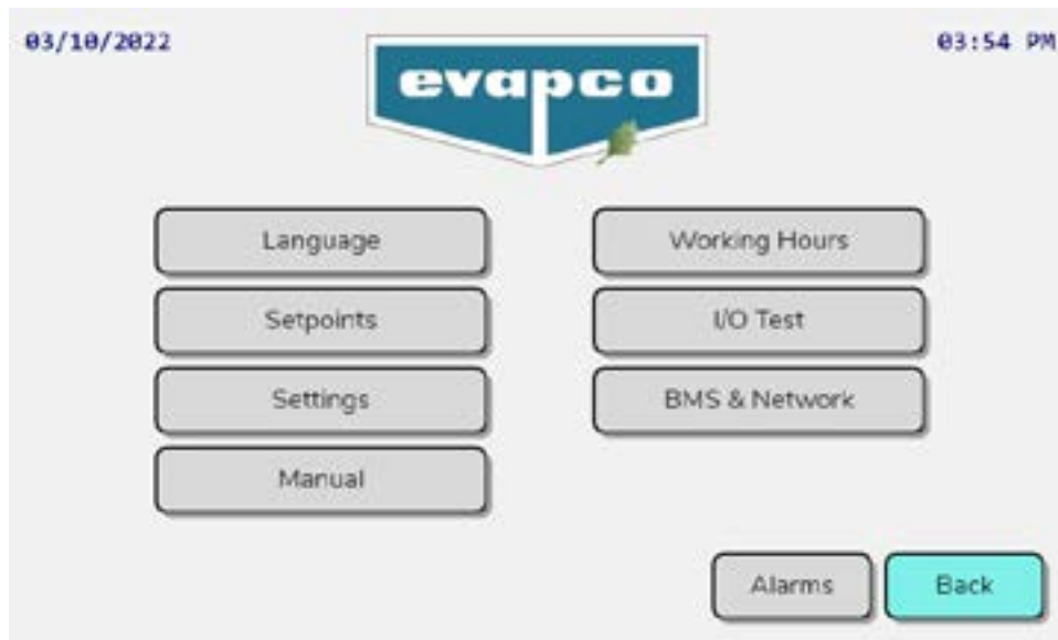
Figure 26 - Service Submenu with Unit Turned Off
