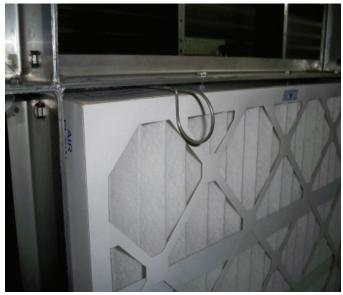
The MERV 14 and 15 final filters are held in place with four spring holding clips or clamps. The MERV 14-15 (95%) filters use a spring clip, fastened to the back flange of the filter frame. Once the tilter is installed, the spring clip should be fastened on the plastic part of the filter. All filters should be installed, if possible, with the pleats vertical.
