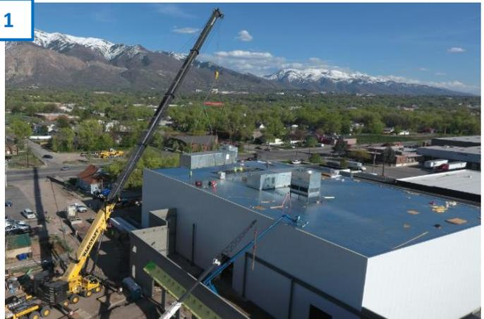
Any additional structural steel needed for roof top packages is minimal if the structural designer incorporates it into the overall building design early in the design development as shown in project Example 1 and Example 2.
