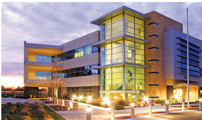
LARGE HVAC APPLICATIONS
