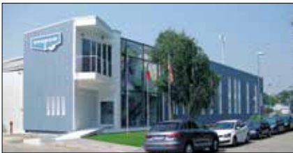
EVAPCO Europe, S.r.l., Milano, Italy
