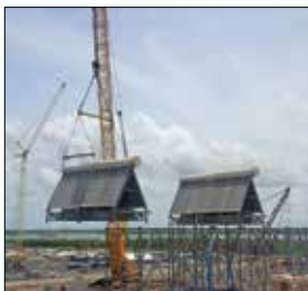
Modularization for efficient installations
