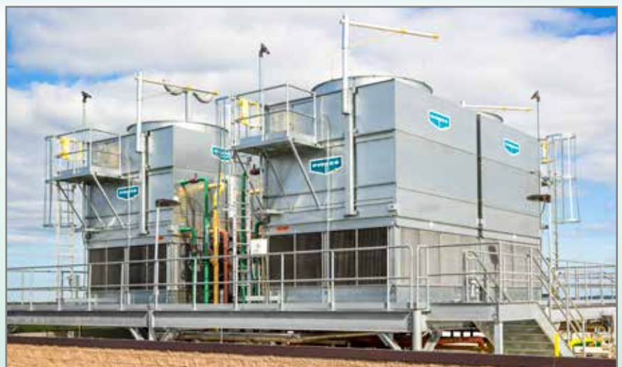
ATC-E Evaporative Condensers with external service platform.
