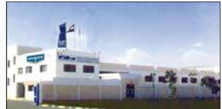
Evap Egypt Engineering Industries Co., Cairo, Egypt
