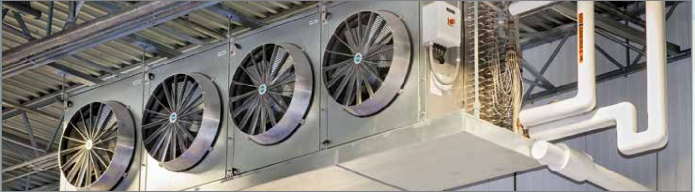
SSTME Evaporator with long-throw adapter
