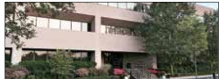
EVAPCO Dry Cooling, Bridgewater, New Jersey
