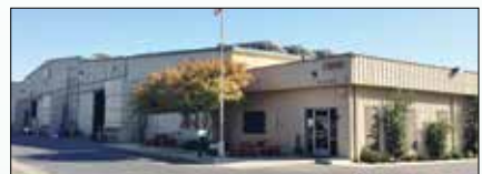
EVAPCO West, Madera, California
