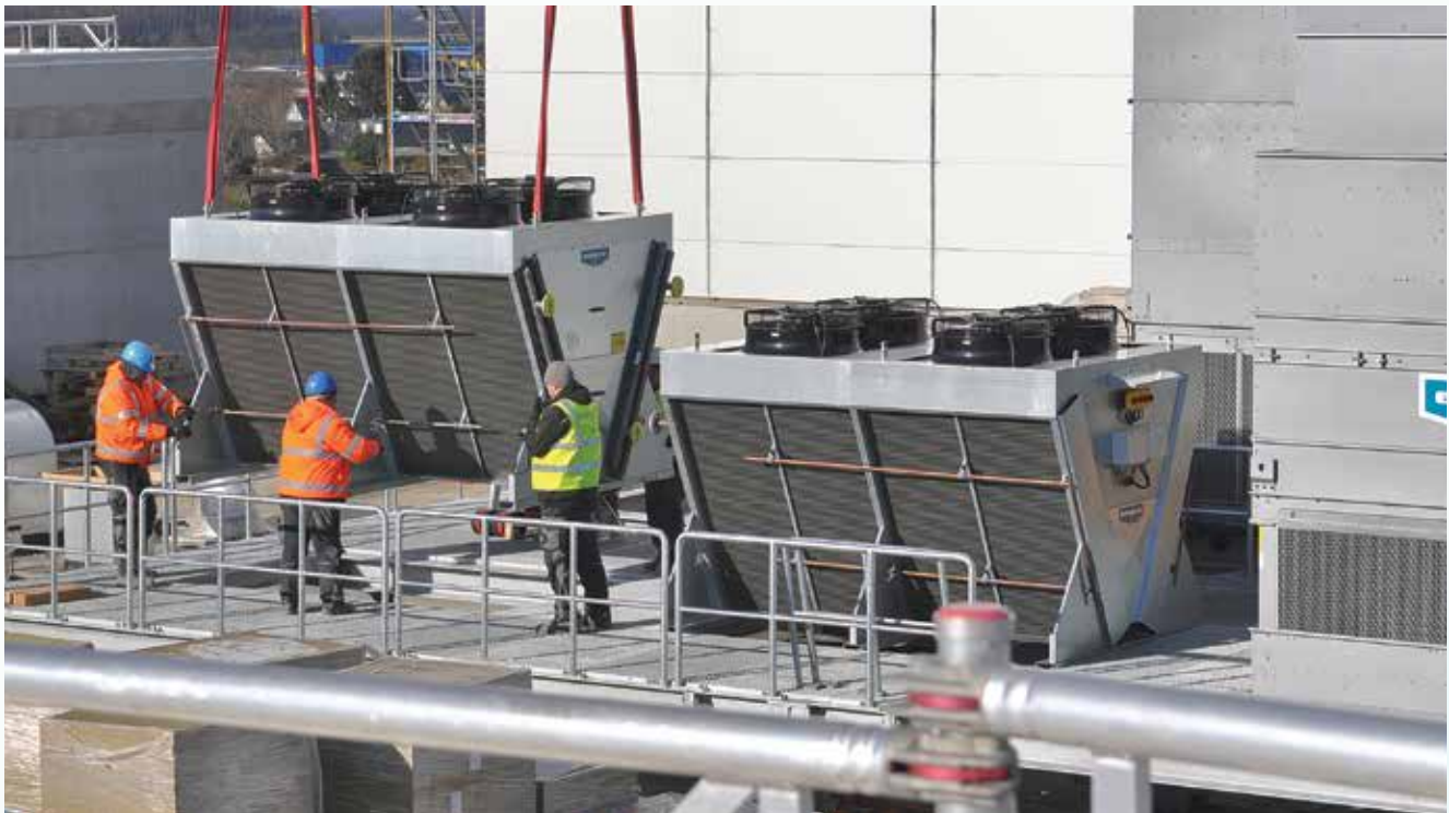
EVAPCO Air Solutions V Series, Germany
