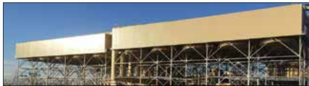
Butterfly arrangement to reduce overall height
