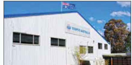
EVAPCO Australia (Pty.) Ltd., Riverstone, NSW Australia
