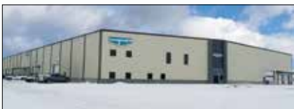
Evapcold Manufacturing, Greenup, Illinois
