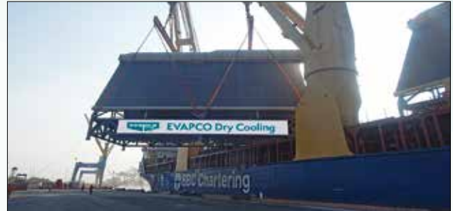
250-ton double fan module transportation
