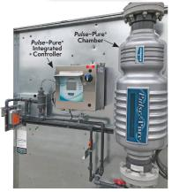
electromagnetic fields to the recirculating water in the PHC-E.
