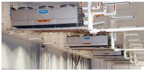
**Evaporators** are built for both ceiling hung and penthouse applications with hygiene in mind.
