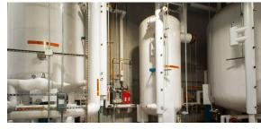
**RVS's recirculators and vessels** keep NH<sub>3</sub> and CO<sub>2</sub> moving efficiently through the system.
