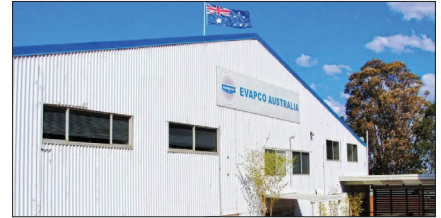
EVAPCO Australia (Pty.) Ltd., Riverstone, NSW Australia
