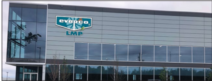
EVAPCO LMP, Laval, Quebec
