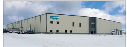
Evapcold Manufacturing, Greenup, Illinois
