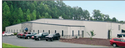
Tower Components, Inc., Ramseur, North Carolina
