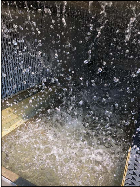
Louver removed for photo
